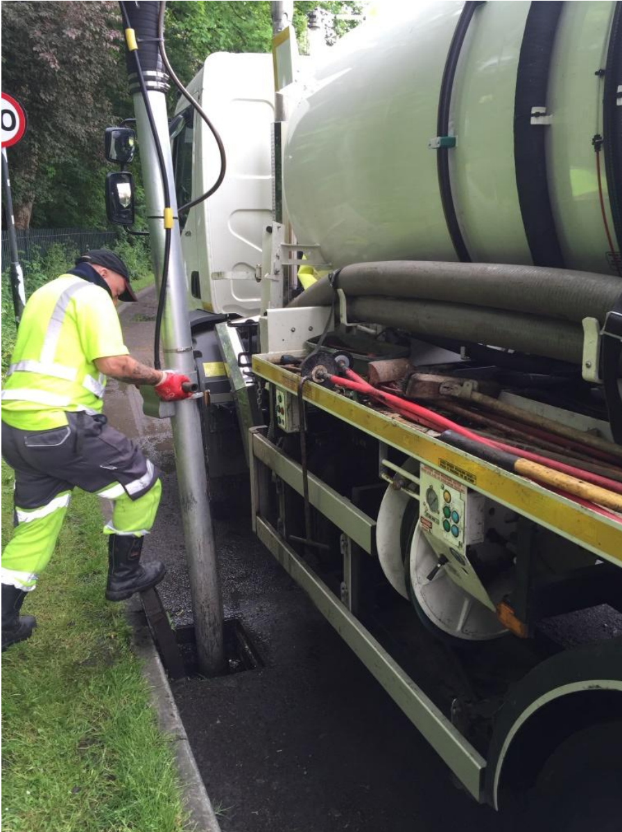
Jetting lorry 11 th June 2016 in Wolfe Avenue
